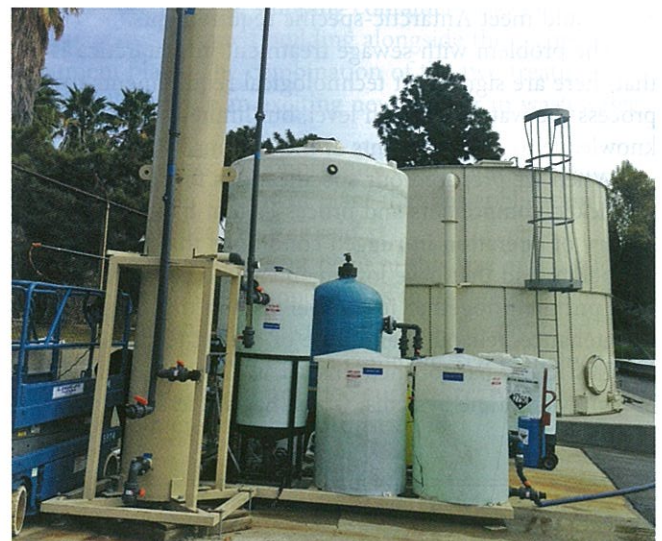
The drinking water plant in Pasadena, California, had the Microvi system installed for nitrate removal as a pilot demonstration.
